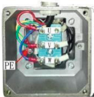
Motor wire connection
